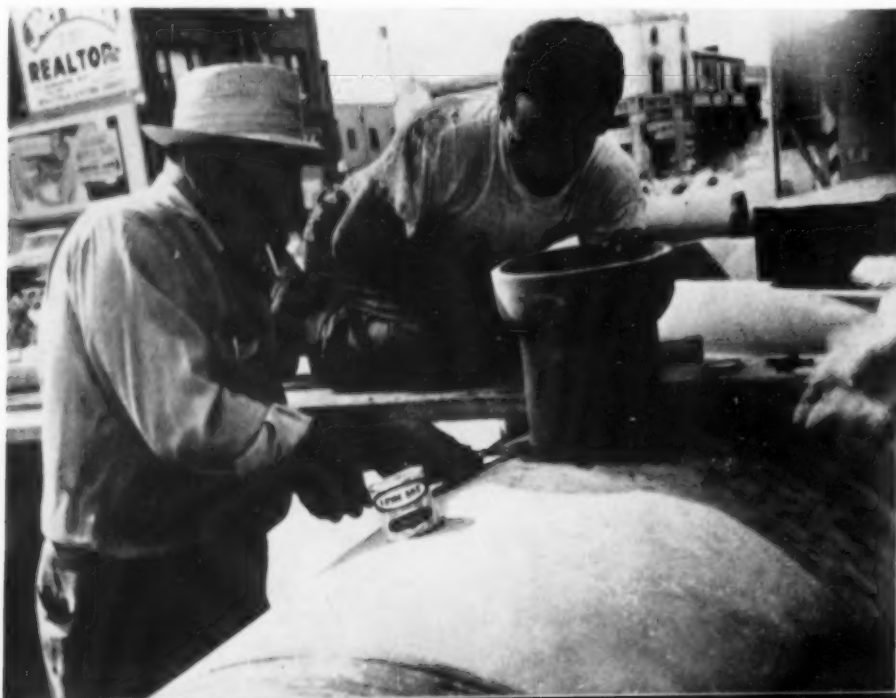
Establishing of a field joint with Epocast 157.
